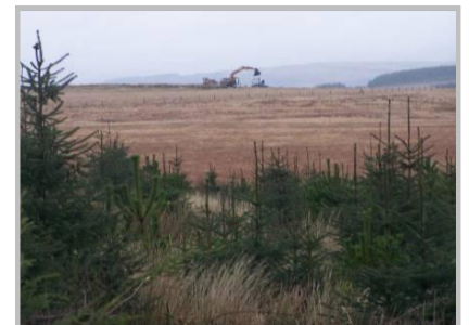
Trial Pit Excavation
