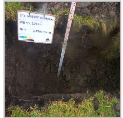
Trial Pit – Detail
