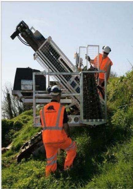
Geotechnical Engineering Ltd has developed a slope climbing rig specifically for the installation of the electrode arrays needed for this process.
