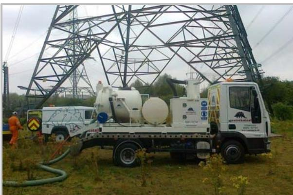
This method eliminates the risk from damage to buried services, whether it be checking known services or pre-drilling at borehole positions.
